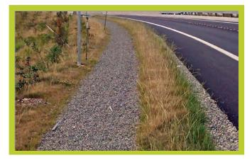
Media filter drains, similar to the one shown here, will filter water running off into Lake Whatcom, removing algaeproducing phosphorus. Because grass is a known source of phosphorus, the filters we install around the lake will not contain the grass strip shown above.
