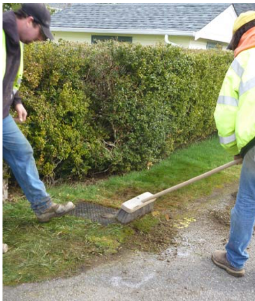
10. The area is cleaned.
