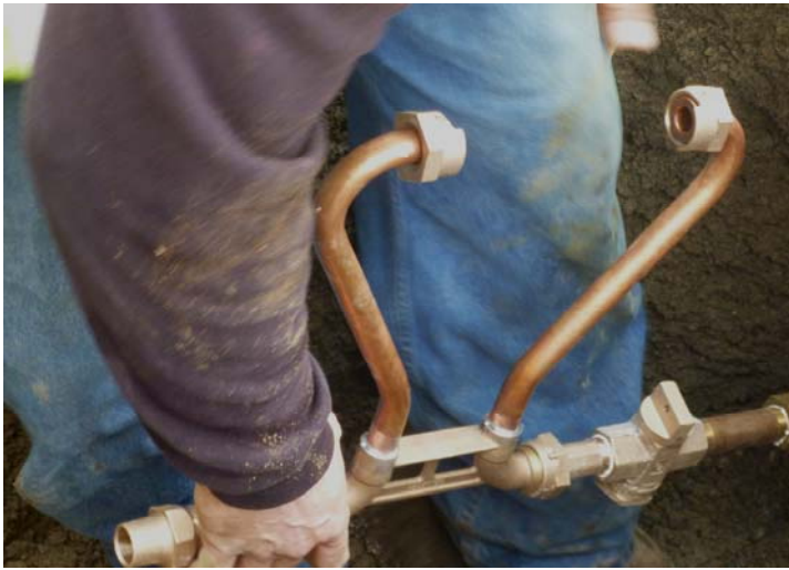
6. The water meter resetter gets installed.
