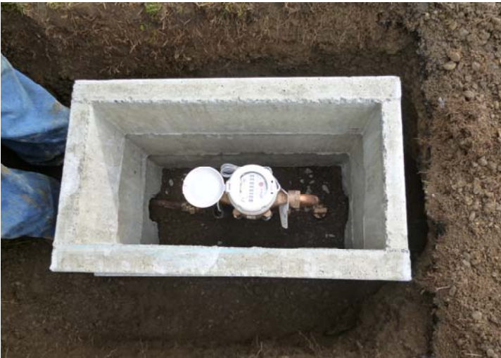
8. The meter assembly box is placed.
