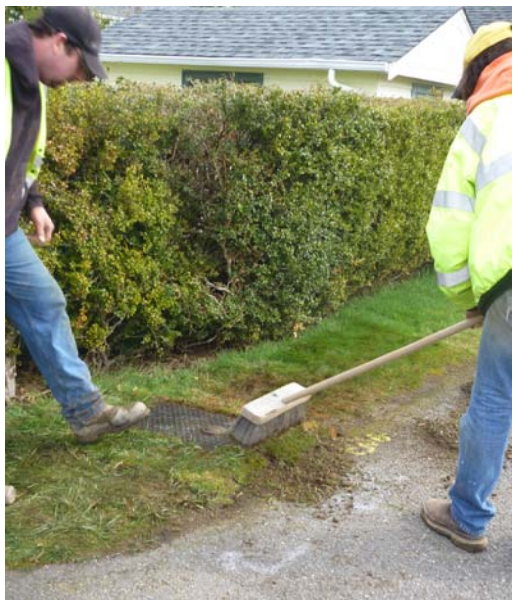
10. The area is cleaned.
