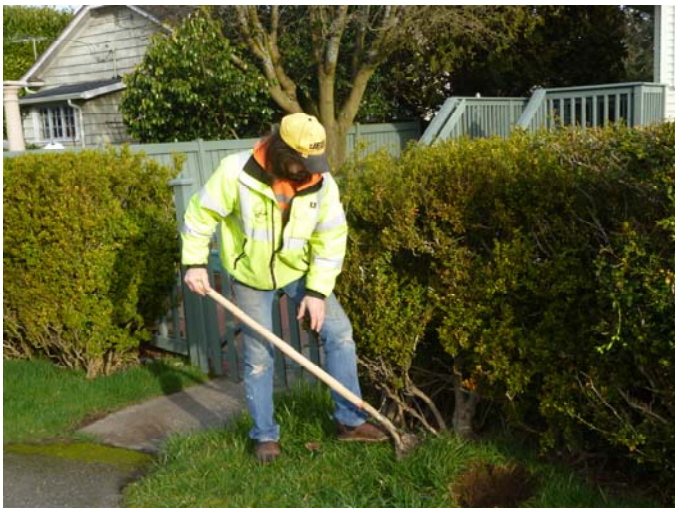
4b. At some sites, crews will dig the hole using shovels.
