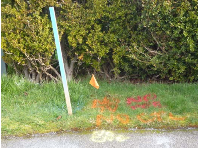
1. Utilities are located in the right-of-way. Several colors of spray paint appear. The blue stake and white paint indicate where water crews will be digging.
