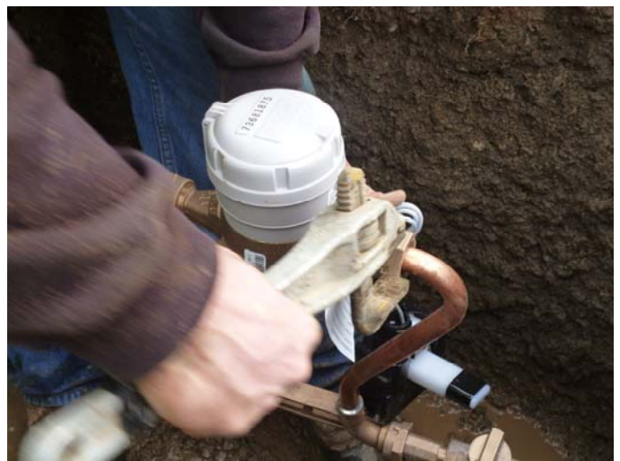
7. Staff installs the water meter and checks for leaks.
