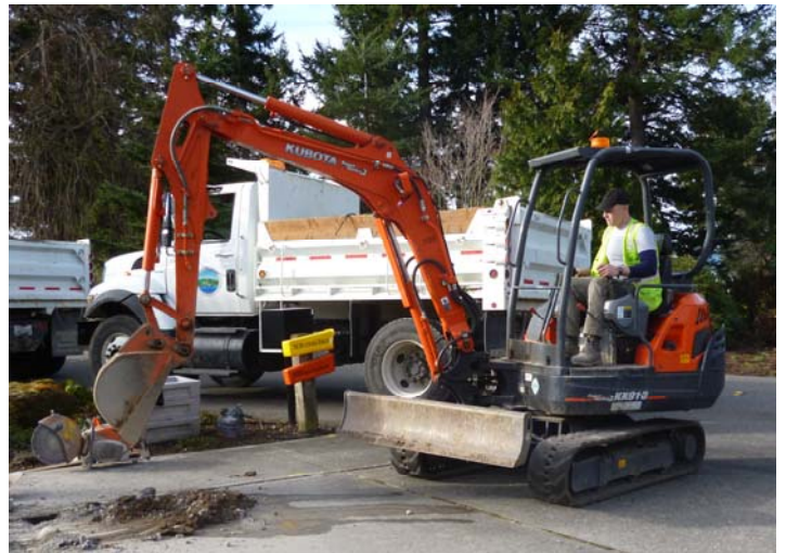
4a. An excavator may dig the hole.
