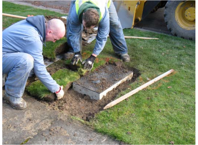
9. A lid covers the box, the hole is filled.
