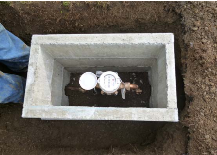
8. The meter assembly box is placed.
