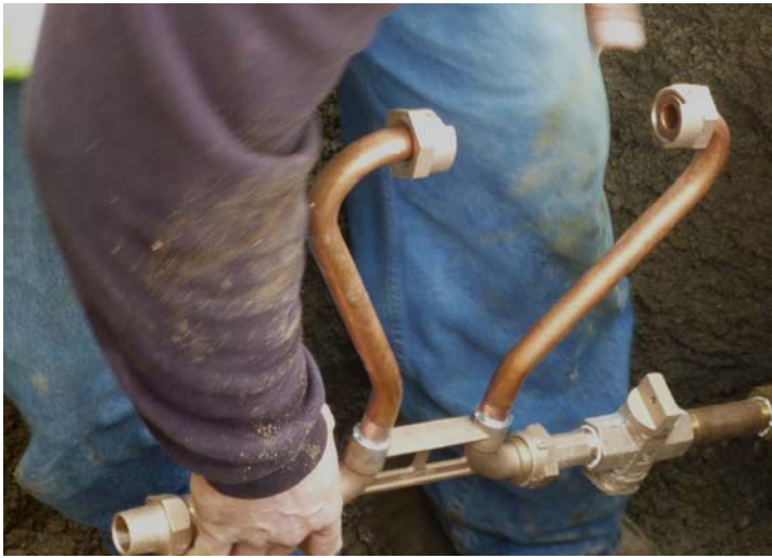
6. The water meter resetter gets installed.
