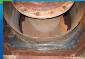
Sand Seal Repair on MHF 1
