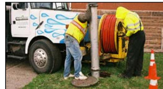
**Wet vaults are large underground storage tanks that use settling for pollutant removal.** Periodic inspection of control structures is needed. Typical maintenance requires the use of a vactor truck.
