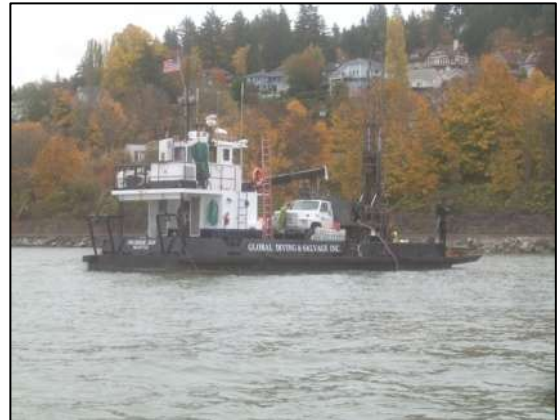
Six geotechnical borings were completed from an anchored barge using a subcontracted truck-mounted drill rig.
