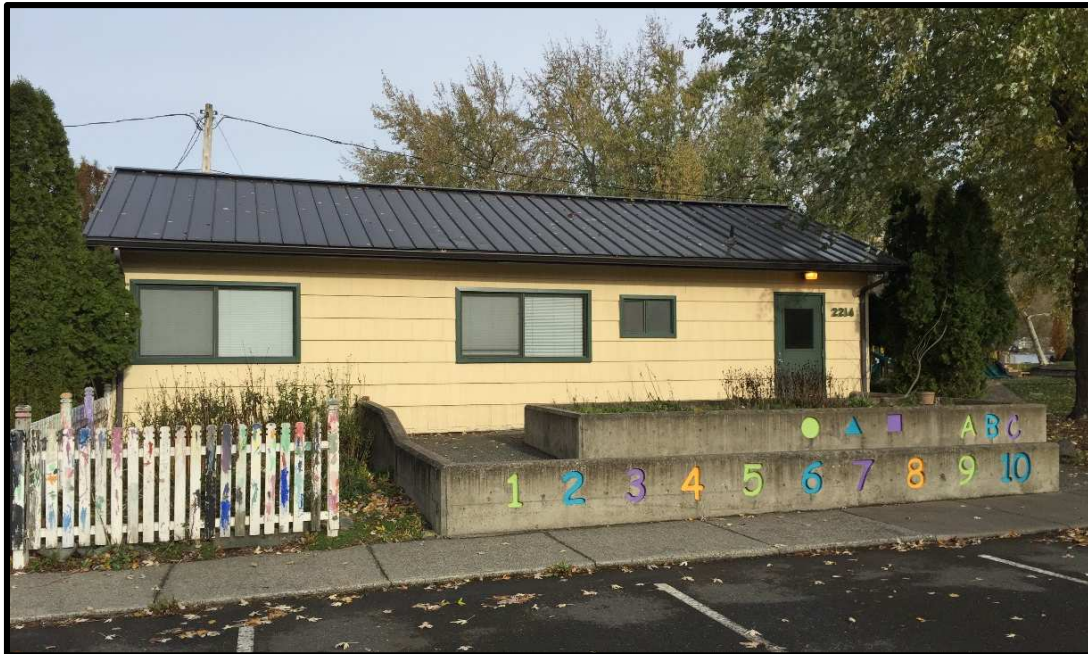
Building exterior from parking lot
