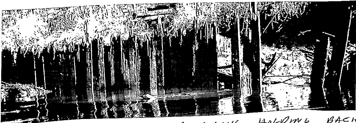
LOOKING N.E. FROM HOLLY ST BRIDGE AT LOW TIDE, OLD CON CRTE/ PILING OBSTRUCTION, OLD PILING ON RIGHT IS BARELY HOLDING BACK THE BANK, WATER DEPTH AT THIS TIDE ABOUT 3-4 FT.
