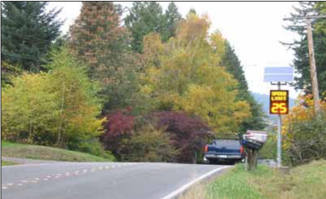
Variable Message Signs on 30th Street collector arterial in South Neighborhood, Bellingham
