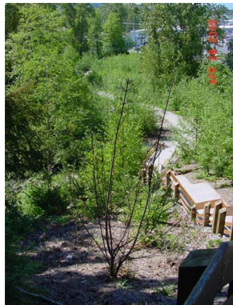
Restoration work along Whatcom Creek, near Woburn Street. WCC crews removed invasive vegetation, stabilized the steep hill, and installed native plants and trees (above). The site after completion of work in 2008 (right).
