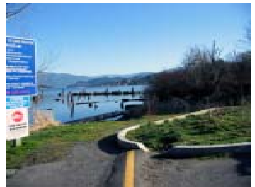
A rain garden doing its job.
