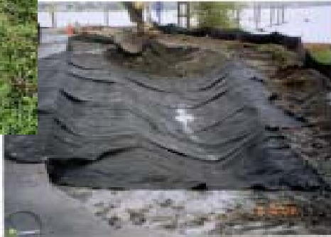
Construction of lower rain garden.
