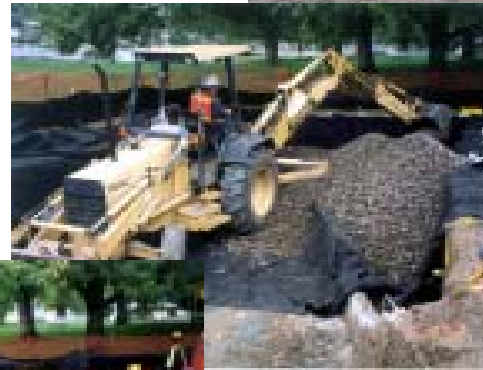
Filter system under construction.
