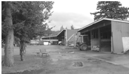
Physical Plant yard
