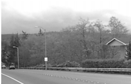
Storm Water Treatment Area (east of apartments)
