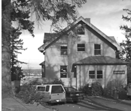
East elevation of Canada House
