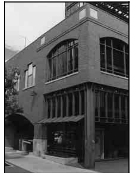
The parking structure (left) incorporates a wrap of retail stores along the street edge. The storefronts are contemporary interpretations of the historic downtown context.
