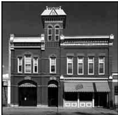
Restoring the firehouse (top photo) to its original condition (middle photo) has helped revitalize a once failing downtown.
