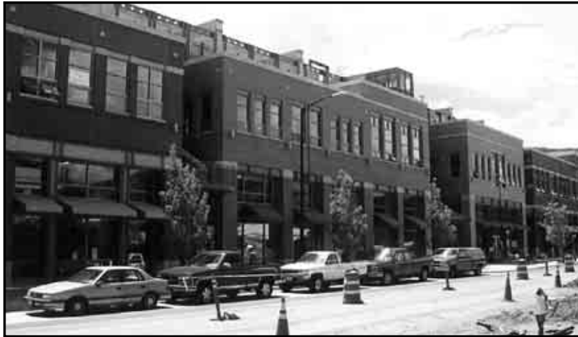
This new infill building is divided into smaller modules in order to relate to the historic buildings across the street.
