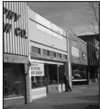
Years later, all original detail had been stripped from the building. (Compare with below.)
