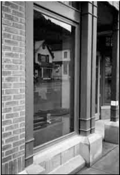
Traditional storefront features—such as a kickplate, display window, transom and recessed entry—are reinterpreted in this new storefront design.
