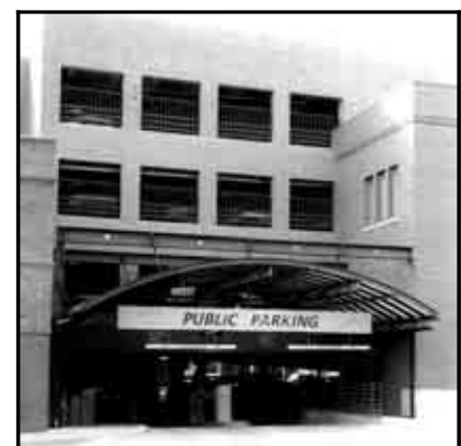
Along one street edge of the parking structure (above left) is the auto-oriented entrance.
