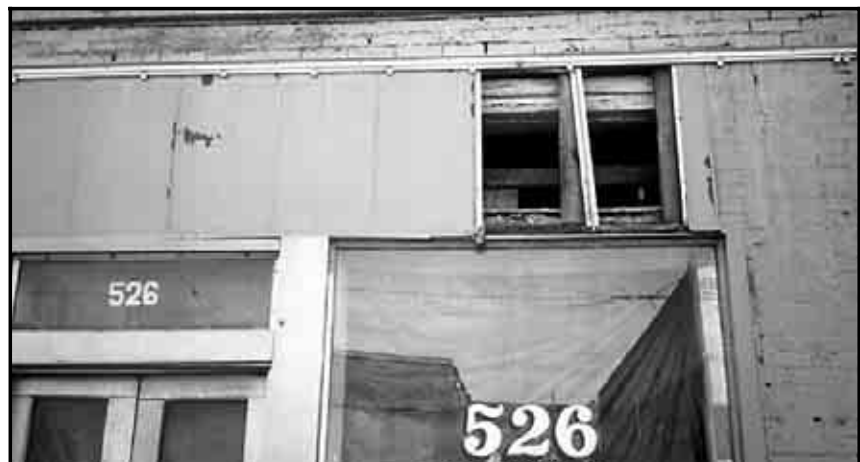
Retain the original shape of the transom glass in an historic storefront. Removing or covering up the transom opening is inappropriate.
