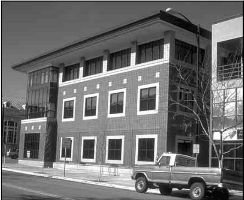
Architectural concrete block combined with brick provides a texture similar to traditional masonry in a contemporary design.
