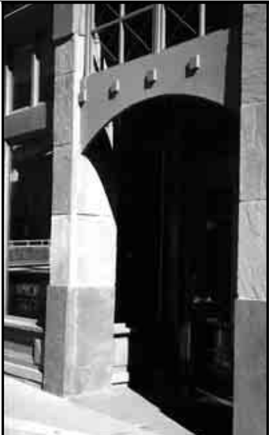
This contemporary interpretation of a storefront (left) includes a recessed entry and transom element.
