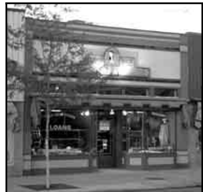
The same building (above) after renovation, exhibits the more classical features of commercial storefronts, including a painted cornice, kickplate, and recessed entry.
