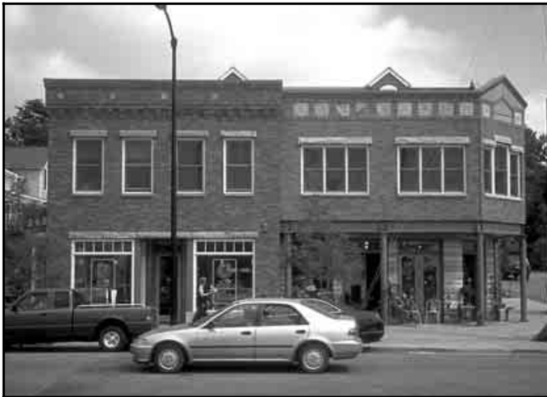
The window sills, moldings, and comices all align on these contemporary infill buildings.
