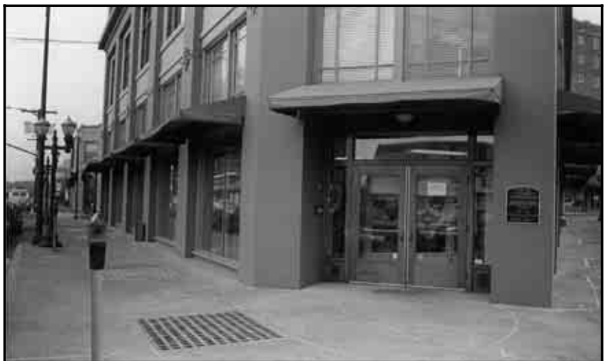
Building entrances should appear similar to those used historically.
