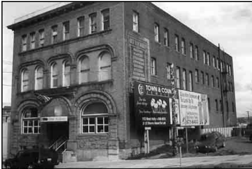
Preserve historic upper story windows.
