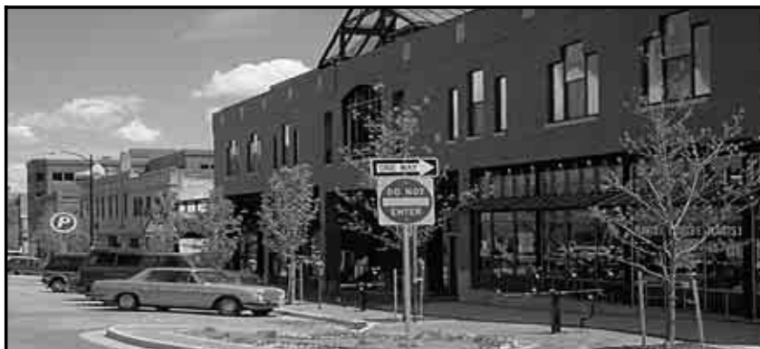
Design a parking structure so that it creates a visually attractive and active pedestrian environment. The series of photographs illustrates this.
