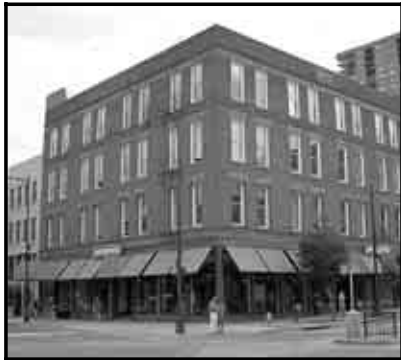
The scale of window and storefront openings on this large infill development helps it relate to the surrounding historic context.
