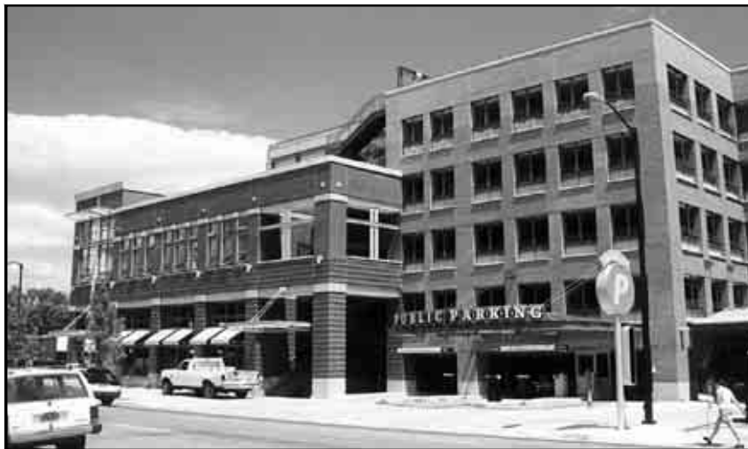
A part of this contemporary infill building (above) is a parking structure which is set back from the front and sides of the retail wrap. The openings in the parking section of the development also utilize “window proportions” similar to those seen historically.
