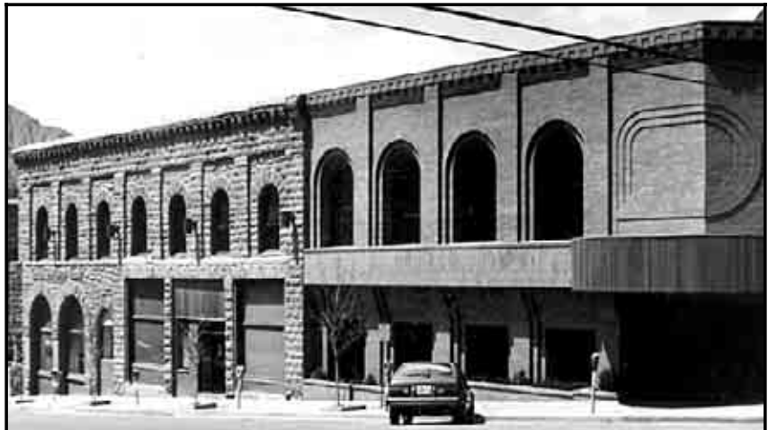
An addition to the side of an existing structure (left) should be compatible in scale and materials, as well as maintaining alignments along the block.
