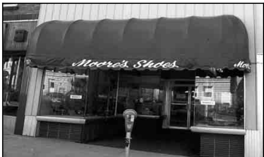
Odd shaped awnings are inappropriate for historical buildings. For example, a bull-nose awning, such as the one seen above, is out of character.
