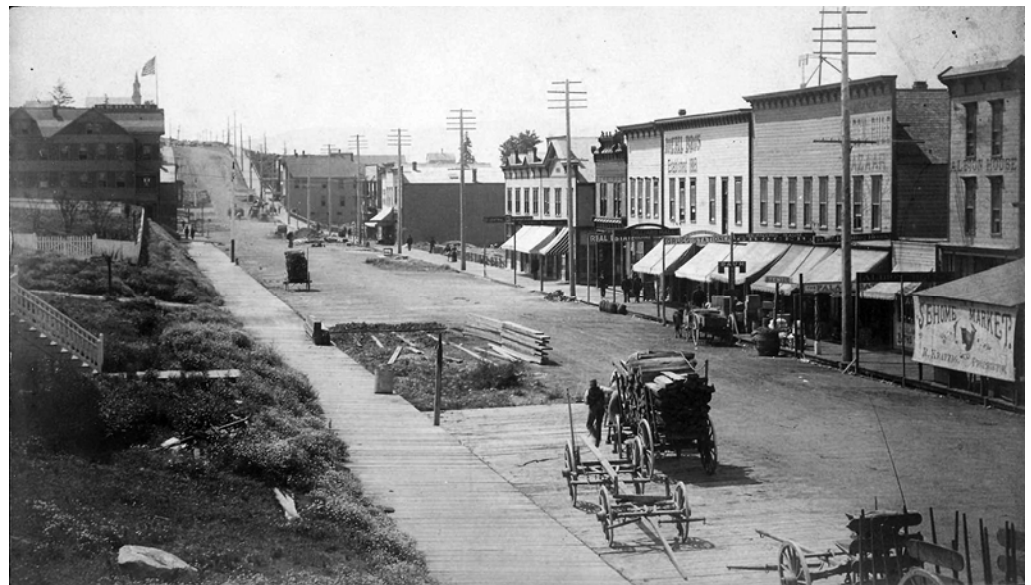
View looking southwest down Elk Street (today's State Street), Sehome, 1890. Elk Street is wood planked -- wagon in foreground is loaded with more planking to fill an exposed area. The Sehome Hotel (upper left) marks the corner of Berry Street. Photo courtesy Whatcom Museum Photo Archives.
