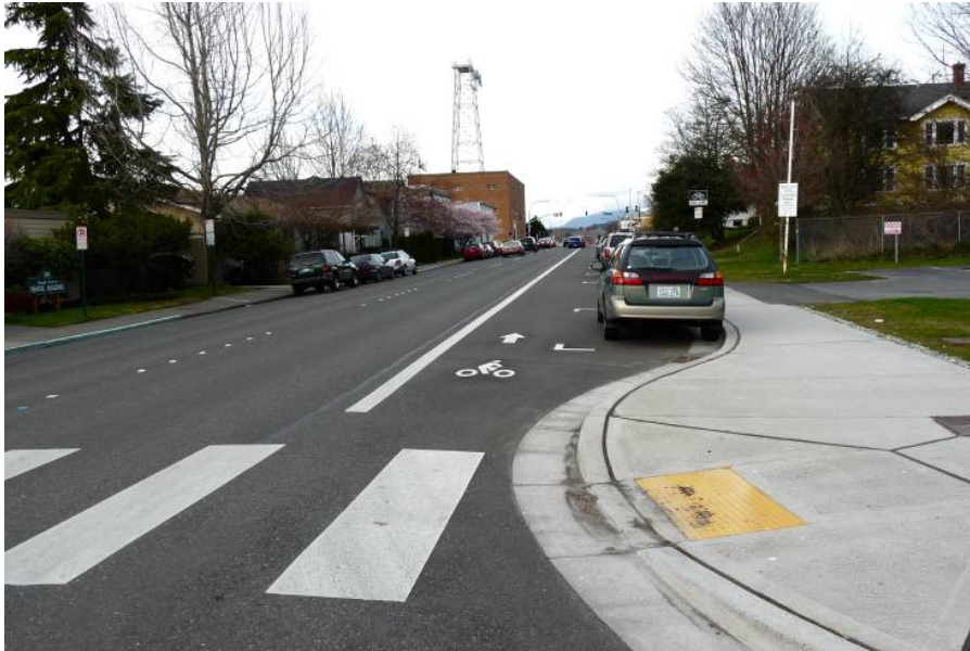
Forest Street is a principal arterial in the Sehome Neighborhood, and has designated bicycle lanes along the south side of Forest Street between Ivy and York Streets. Photo courtesy Joy Keenan.
