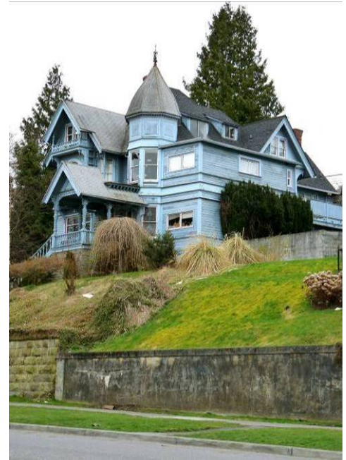
The Morse House on Garden Street is listed on the National Register of Historic Places. Originally built as a single-family residence, the building has been adaptively used over time as a bed and breakfast and as multi-family housing. Photo courtesy Joy Keenan.
