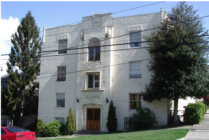
The historic Alamo Apartments on Maple Street and Garden Street. Photo courtesy Joy Keenan.
