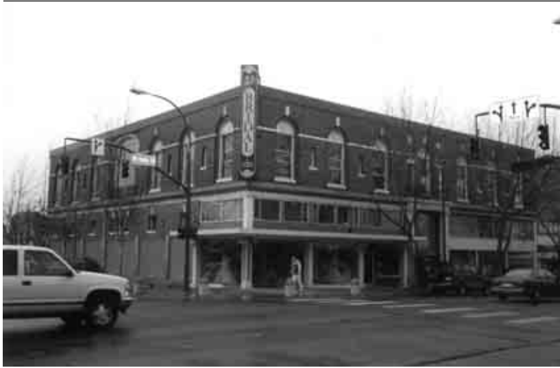
The intersection of Holly at Commercial is an example of where a type A intersection would be appropriate.
