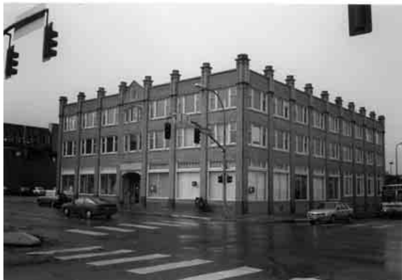
The intersection of Magnolia at State is an example of where a type C intersection improvements might be appropriate.
