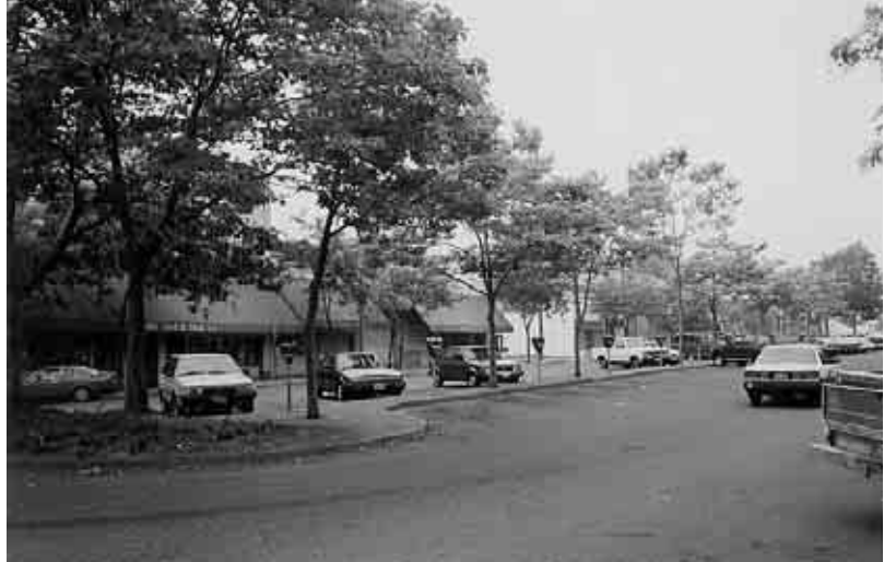
As a means of enhancing the pedestrian connection along Railroad Avenue, the center median should be widened.
