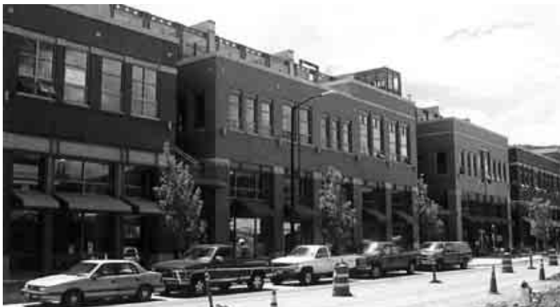
Parking facilities should be designed to reinforce the traditional commercial building context of downtown. This design for a new garage recently completed in Boulder, Colorado, includes a "wrap" of retail and office space that animates the street edge.
