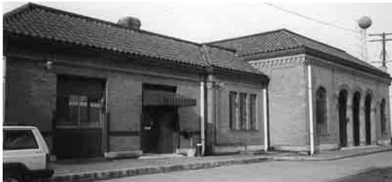
The railroad dept, at Holly and E Streets, is an important landmark in the City Center. (#4)
