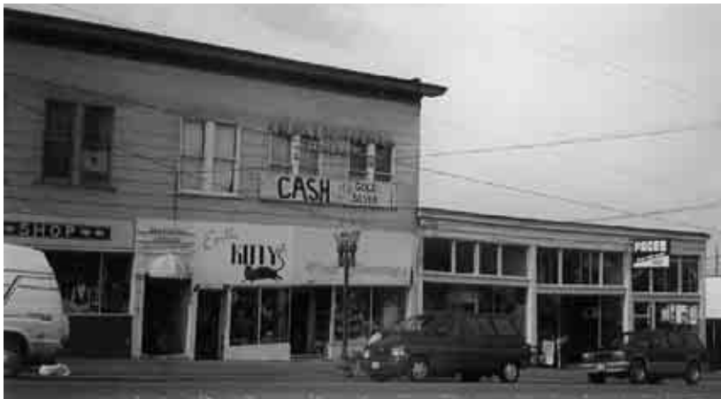
The upper portion of Old Town exhibits traditional storefronts that align at the sidewalk edge.
