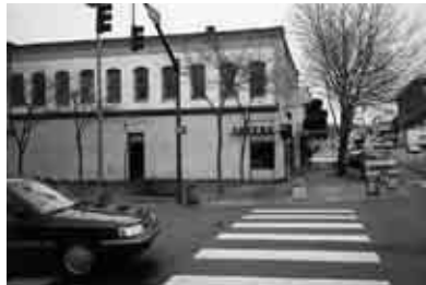
The former Flame Tavern site is being redeveloped with ground floor commercial and three floors of dwelling units.
