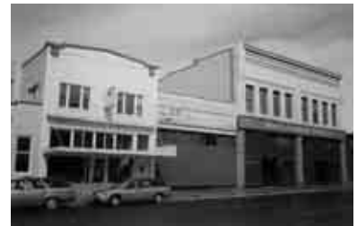
The Morse hardware property.
