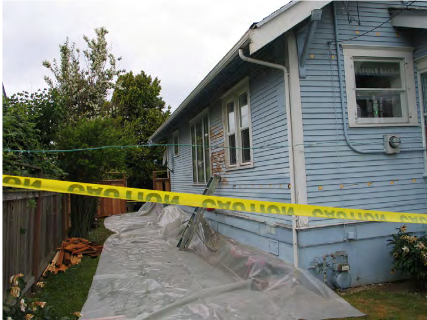
Home Rehabilitation on House with Lead-Based Paint
